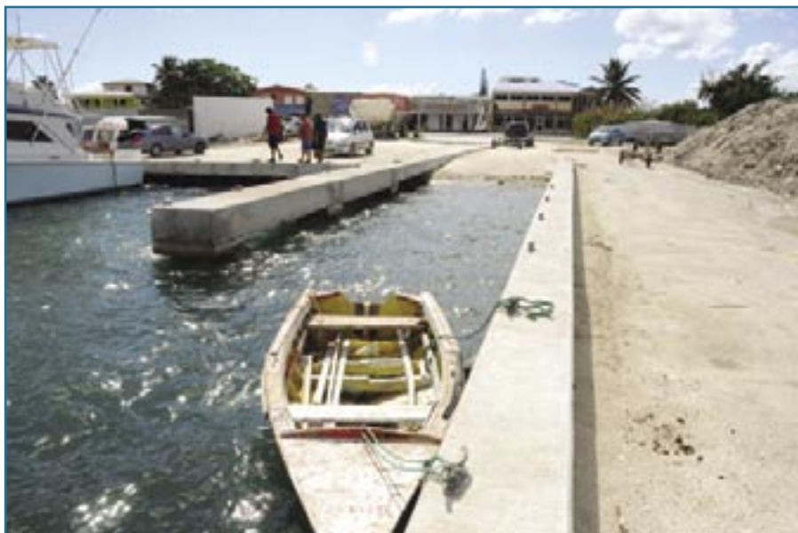
The new fisherman's jetty in the Simpson Bay Lagoon.
