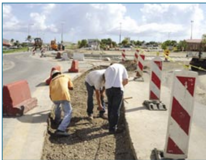
The new road is almost finished
